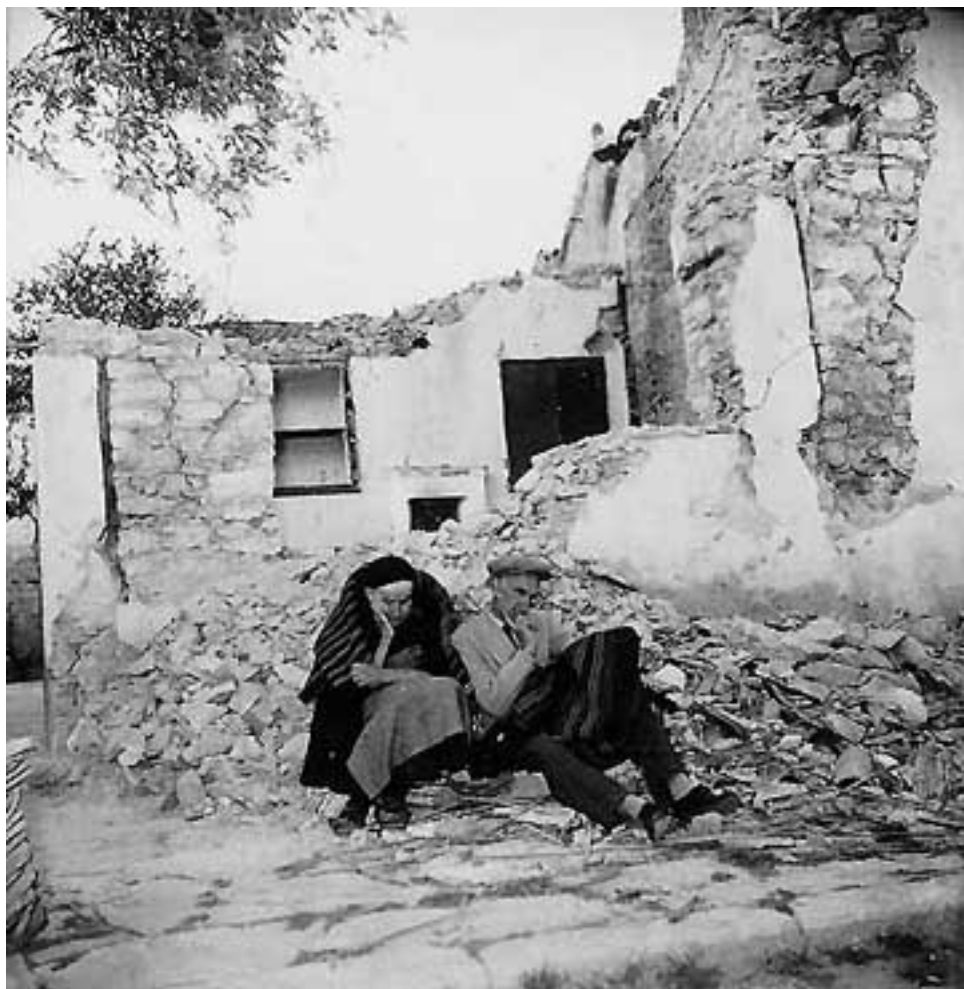
After the earthquakes ..., Archive DIKI
