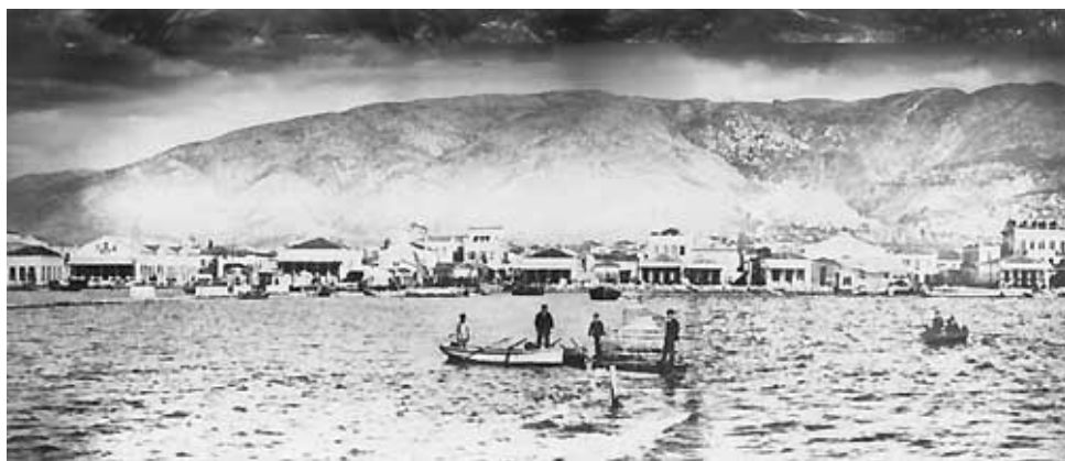
Wooden quay in the port of Volos, 1894. Photograph by Stournaras, Town Hall.
