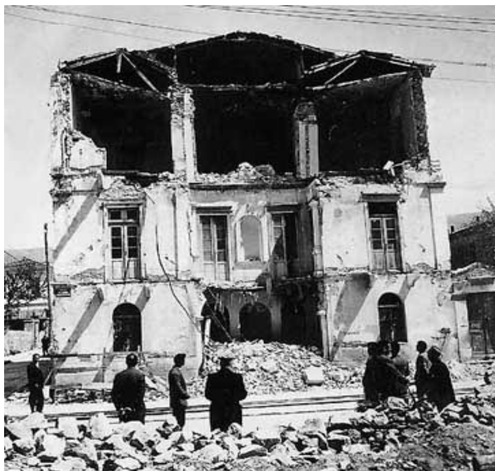
After the earthquakes ..., Archive DIKI
