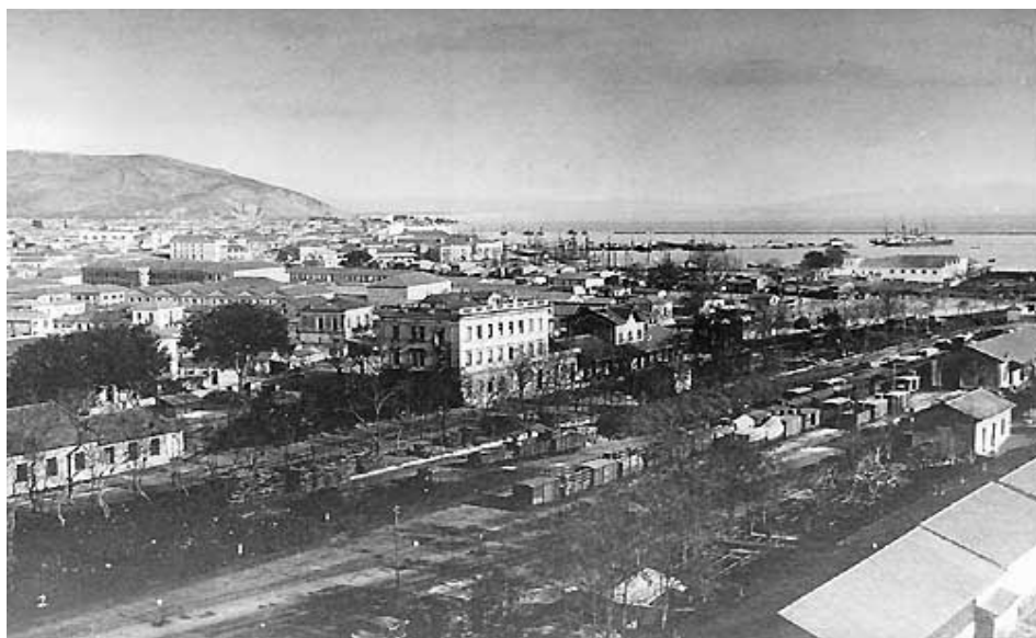
Panoramic view of the railway station, ca. 1940. Archive Zimeris, DIKI.
